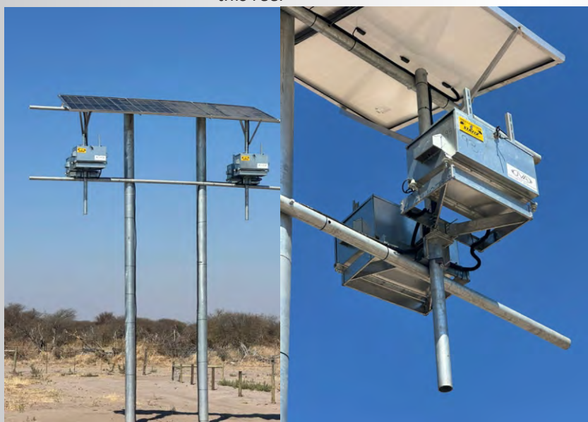
Game elephant fence in the pans in Botswana with an interesting floating type fence on the river crossings. Note our pole mount shock boxes - the fence is powered by a Stafix X18.
