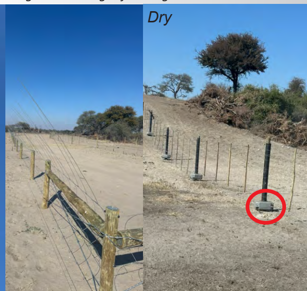
Game elephant fence in the pans in Botswana with an interesting floating type fence on the river crossings. Note our pole mount shock boxes - the fence is powered by a Stafix X18.
