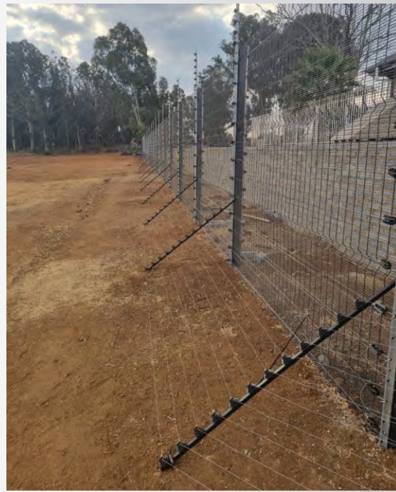
12-line Wall-top brackets being used to create an anti-dig apron
