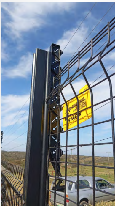
A little bit of improvisation – mounting the plastic bracket to clearview
