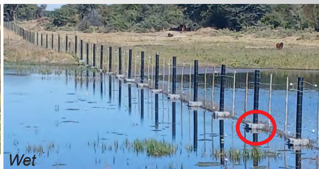
Clever use of floating posts to raise and drop the fence during tides and light flooding
